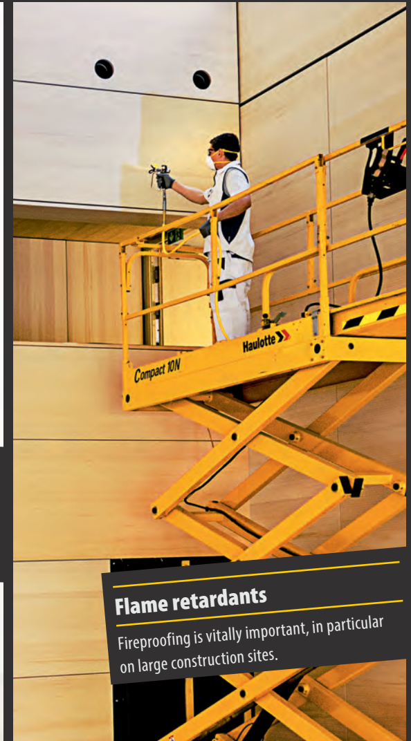
Spraying textured plasters indoors The machine application of fillers saves effort and time. It is the economic, efficient, intelligent way to work on-site.
